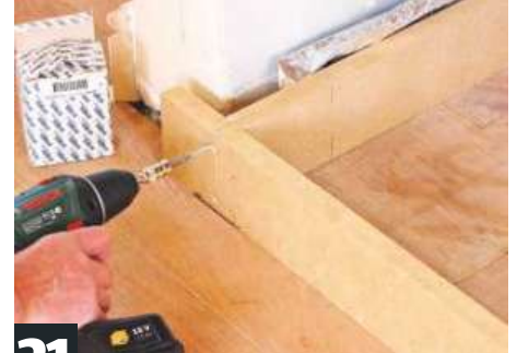
21 To finish flush with skirting, base of cupboard sits on plinth. Build from MDF and screw sections together
